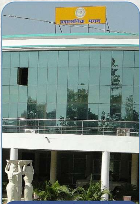
Administrative Building ANDUA&T, Ayodhya
